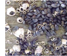
Barnacles and Mussels on Pier Piling
